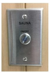
This switch cannot function as a control. It has to be connected to the system with another control.
